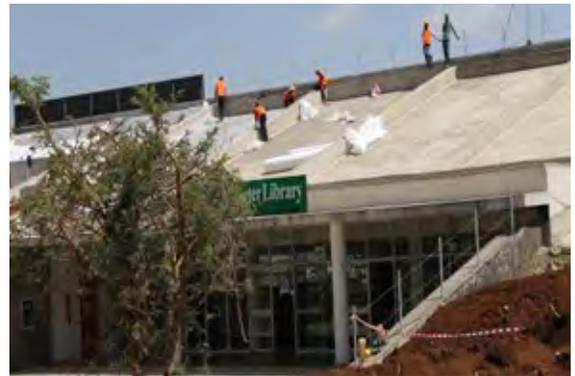
ducted during the period. Two layers of polyethylene were applied on the roof of the library to protect water from seeping into the roof. Red soil was spread on the rooftop for planting grass. The work was undertaken with good plan and the library cover has now been completed, restoring the beautiful scenery of the campus.
