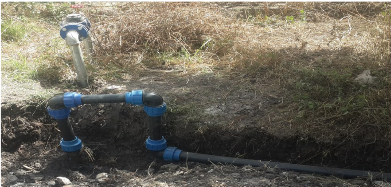
The new water supply line extension
