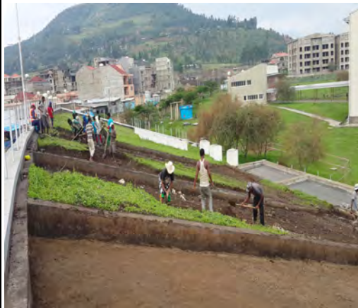
Library roof repair underway
