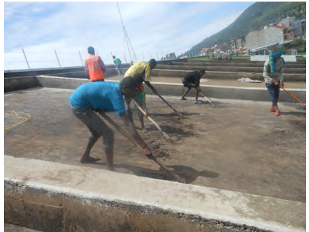
Library roof repair progresses further
