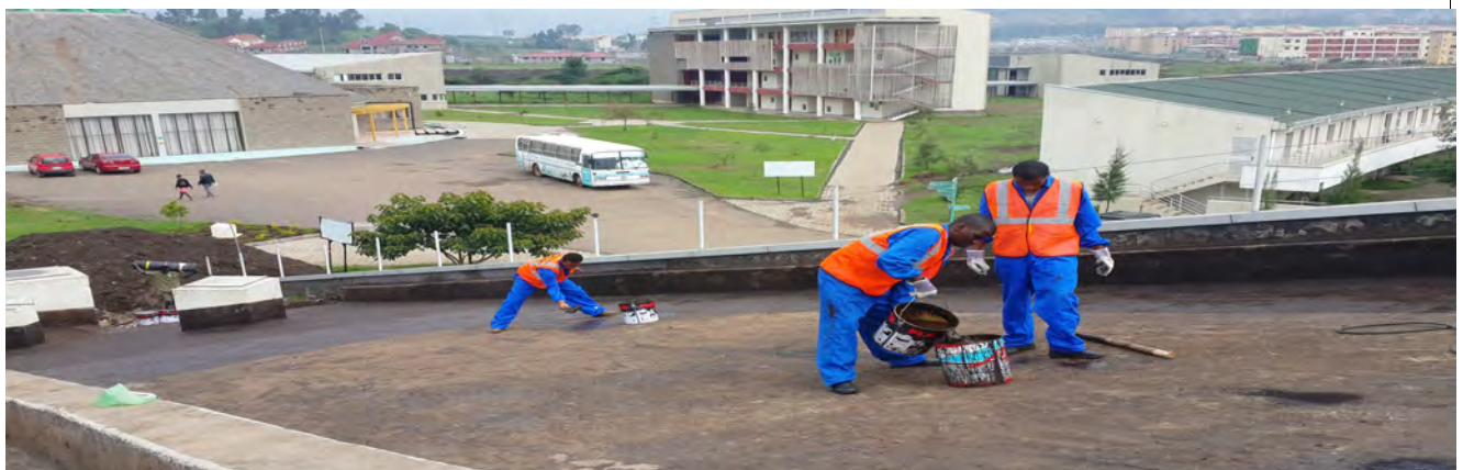
Preparing for waterproofing
