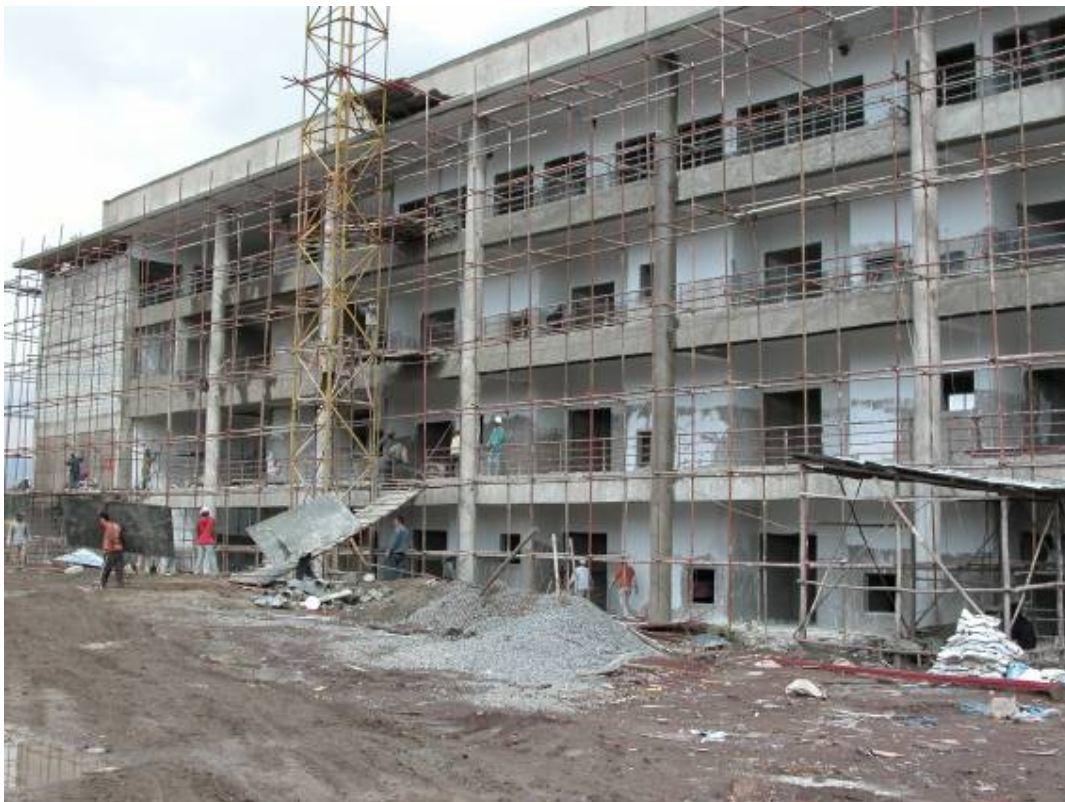
Classroom F (second classroom building)
