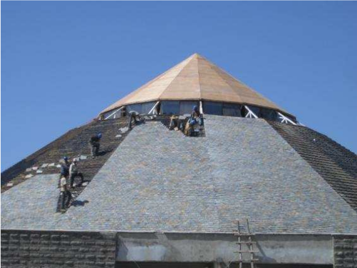
Started on the natural oxidized slate roofing for the auditorium.
