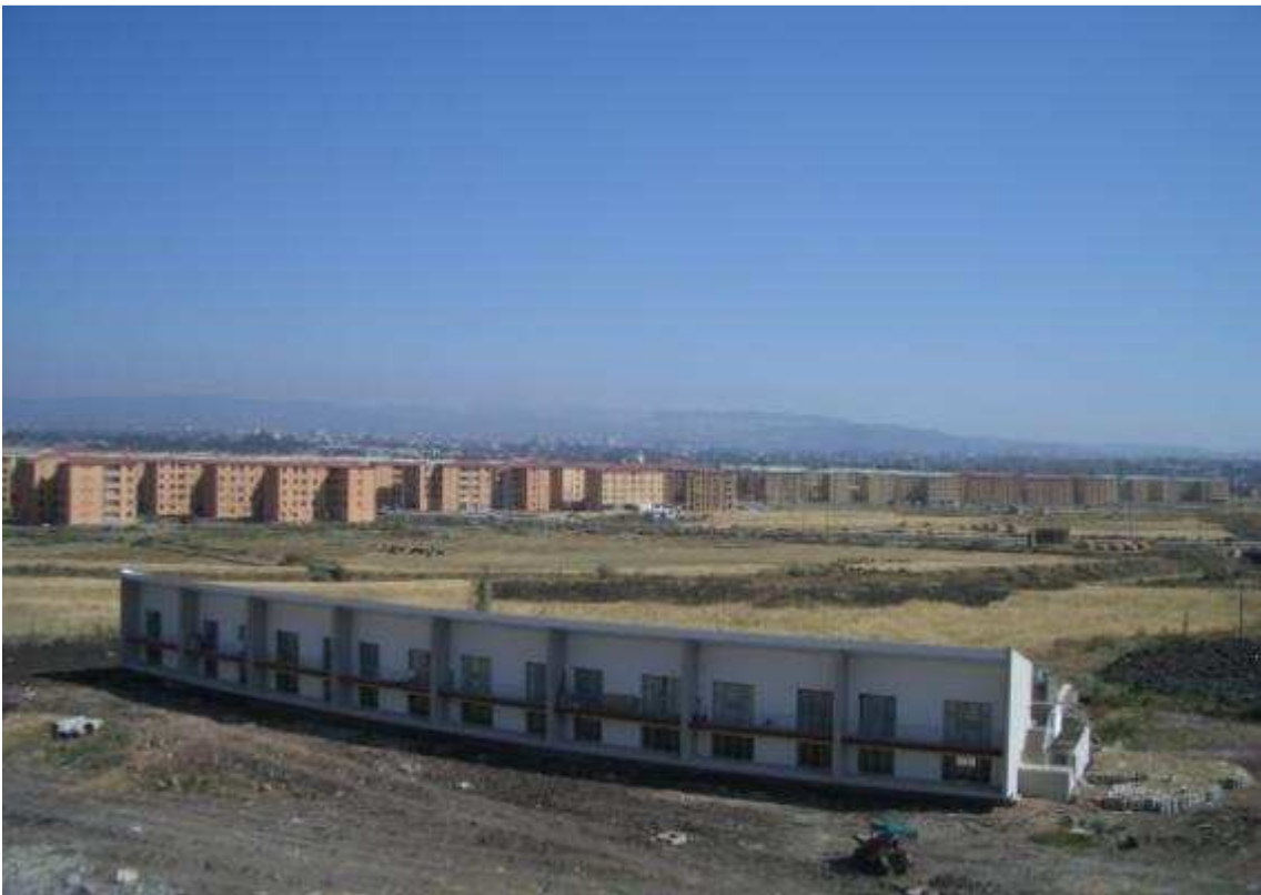
The staff residence, already in use.
