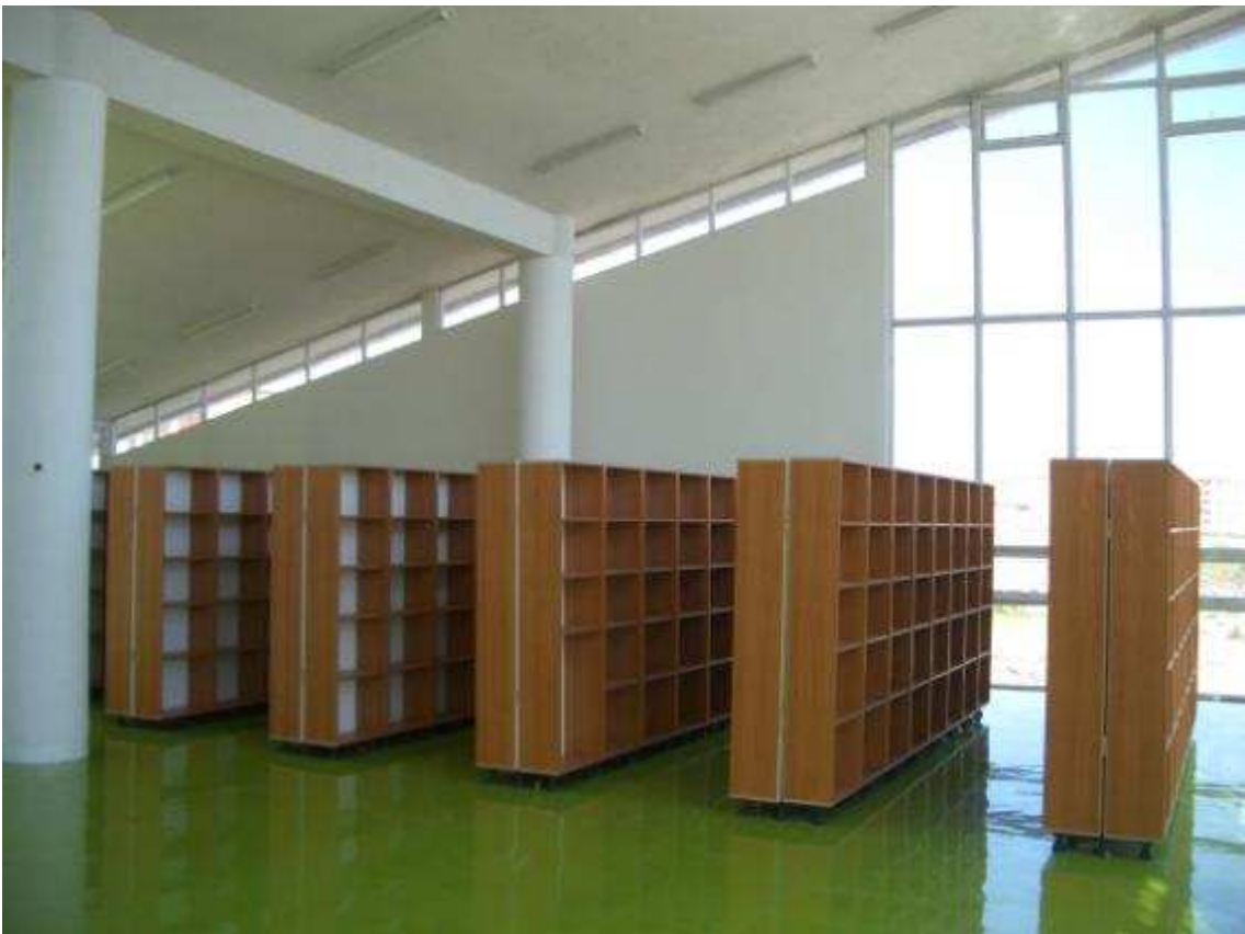
The shelves are being put in place.
