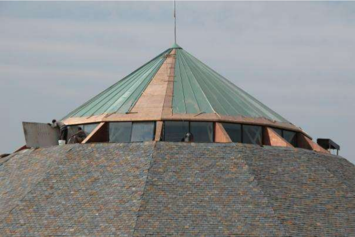
Multi-purpose hall with slating and top of copper.
