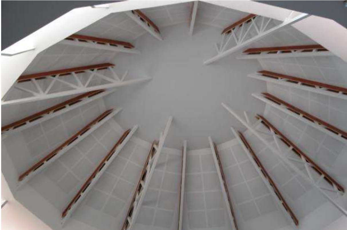
The acoustic ceiling with dome in the Multi-purpose hall.
