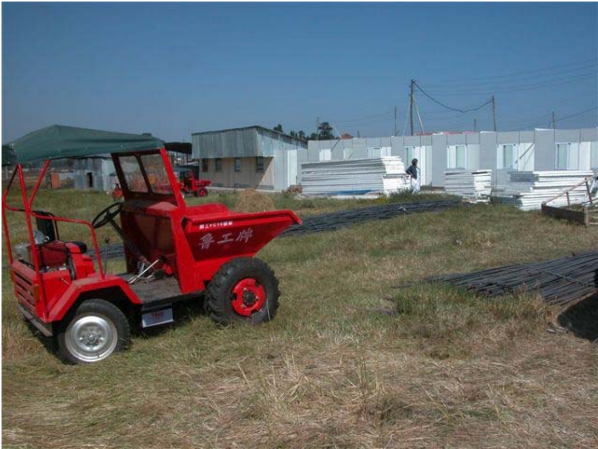
Temporary offices under construction; in the foreground a concrete dumper
