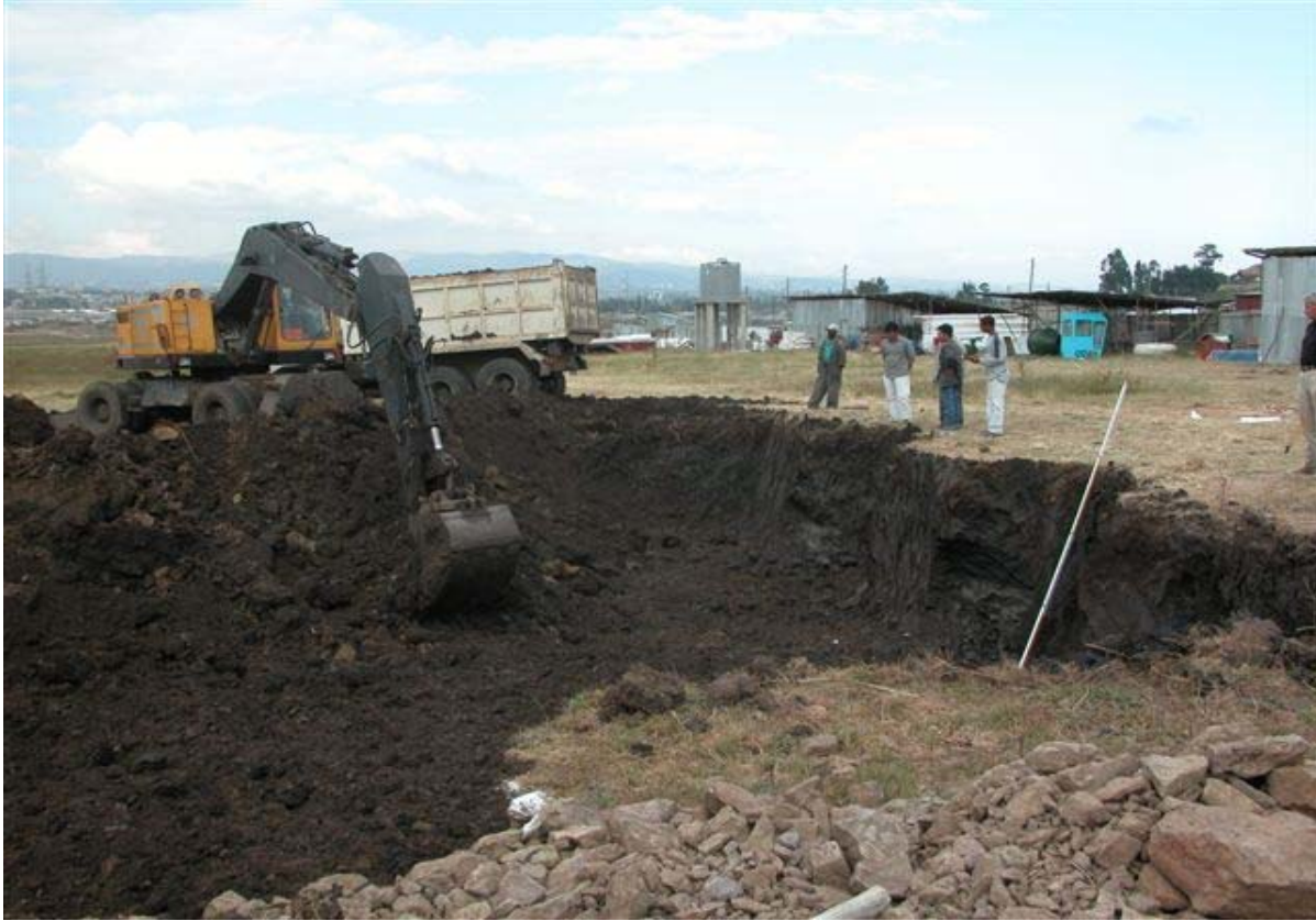
Excavation to the Service Center has begun.
